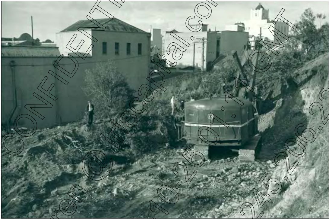
FIGURE 2.2 1961 photograph showing site clearing and excavation works for the construction of the King Street Car Park. Note the depth of excavation through the natural soil profile of the site - shown as pale deposits on the right of photograph. King Street is located outside the photograph to the right
