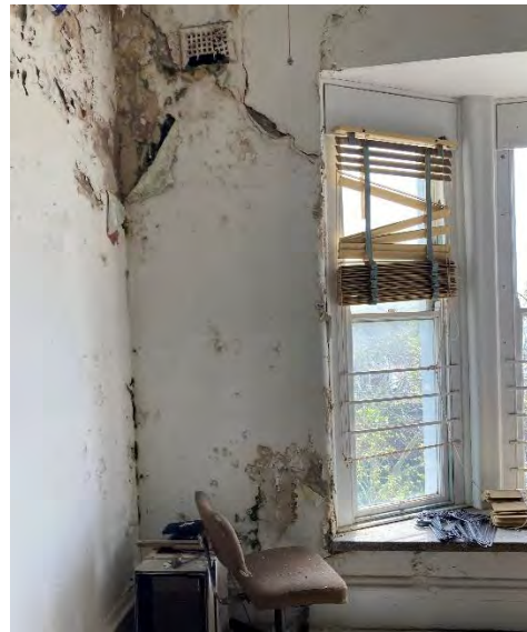
Figure 45: Dampness along the internal walls with peeled-off plaster.
