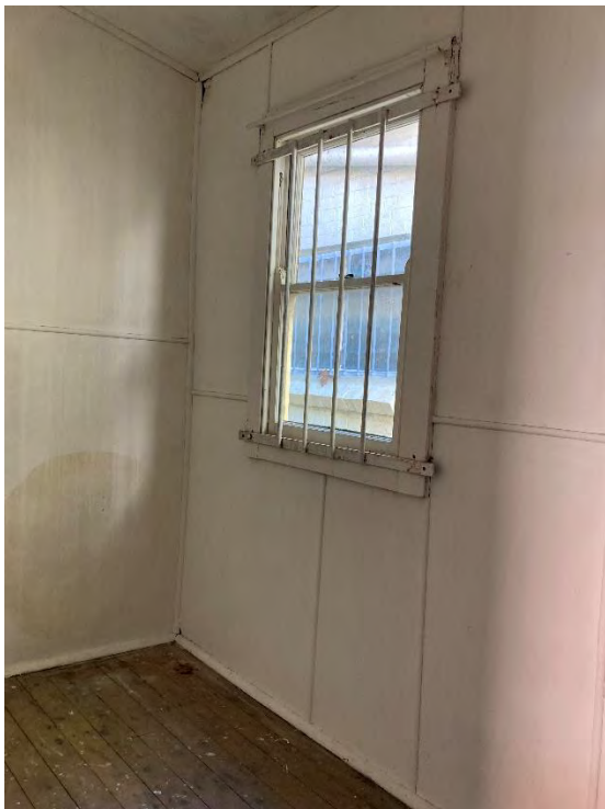
Figure 38: Timber framed single-hung windows with metal grill.
